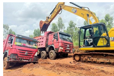
Excavator loading Sala Pressure tipper trucks.
