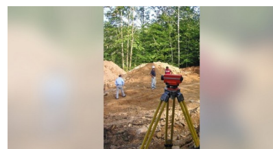
Automatic level set up on an earthworks site.
