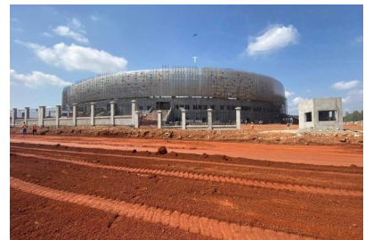
Access road earthworks beside a stadium under construction.
