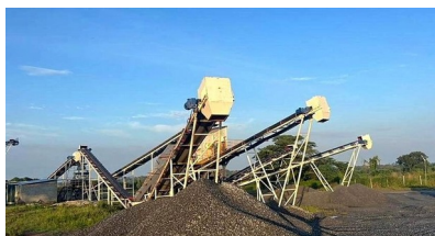
Crushing and screening plant with aggregate stockpile.
