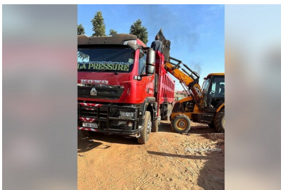
Backhoe loader loading a red tipper truck.
