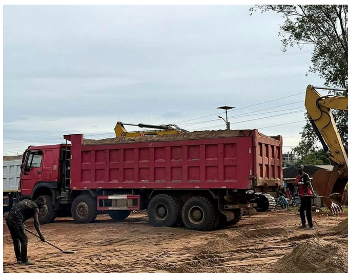
Sala Pressure tipper truck being loaded with sand on site.
