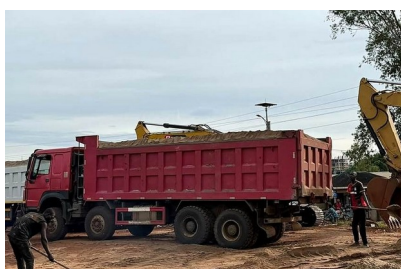
Tipper being loaded with sand.
