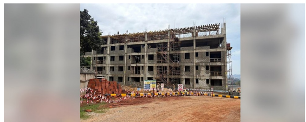
Multi-storey building with concrete frame, block walling and scaffolding.
