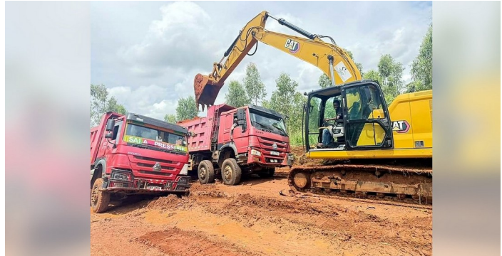
Excavator loading Sala Pressure tipper trucks on an earthworks site.
