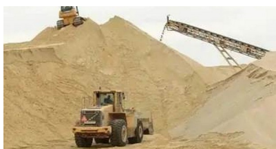
Wheel loader working on a sand stockpile.
