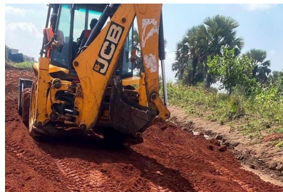
Backhoe loader grading an access road.
