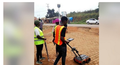
Ground penetrating radar (GPR) survey in progress.
