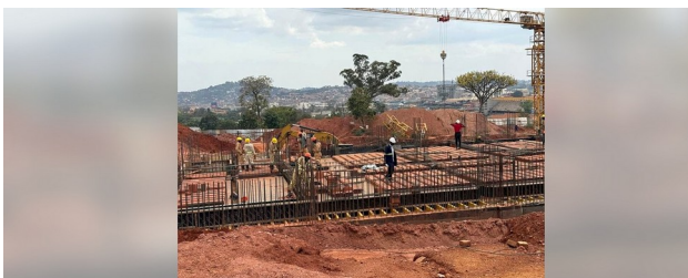
Foundation and slab works with excavator and tower crane.
