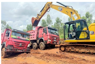
Excavator loading tipper trucks.
