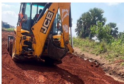
Backhoe loader at work on a road.
