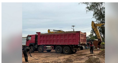
Red tipper truck being loaded with sand.
