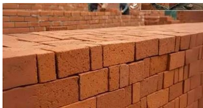
Burnt clay bricks laid in a wall.
